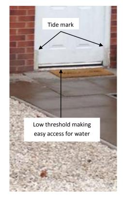
Figure 6: Example of tide mark and low threshold on Bakewell Drive.
