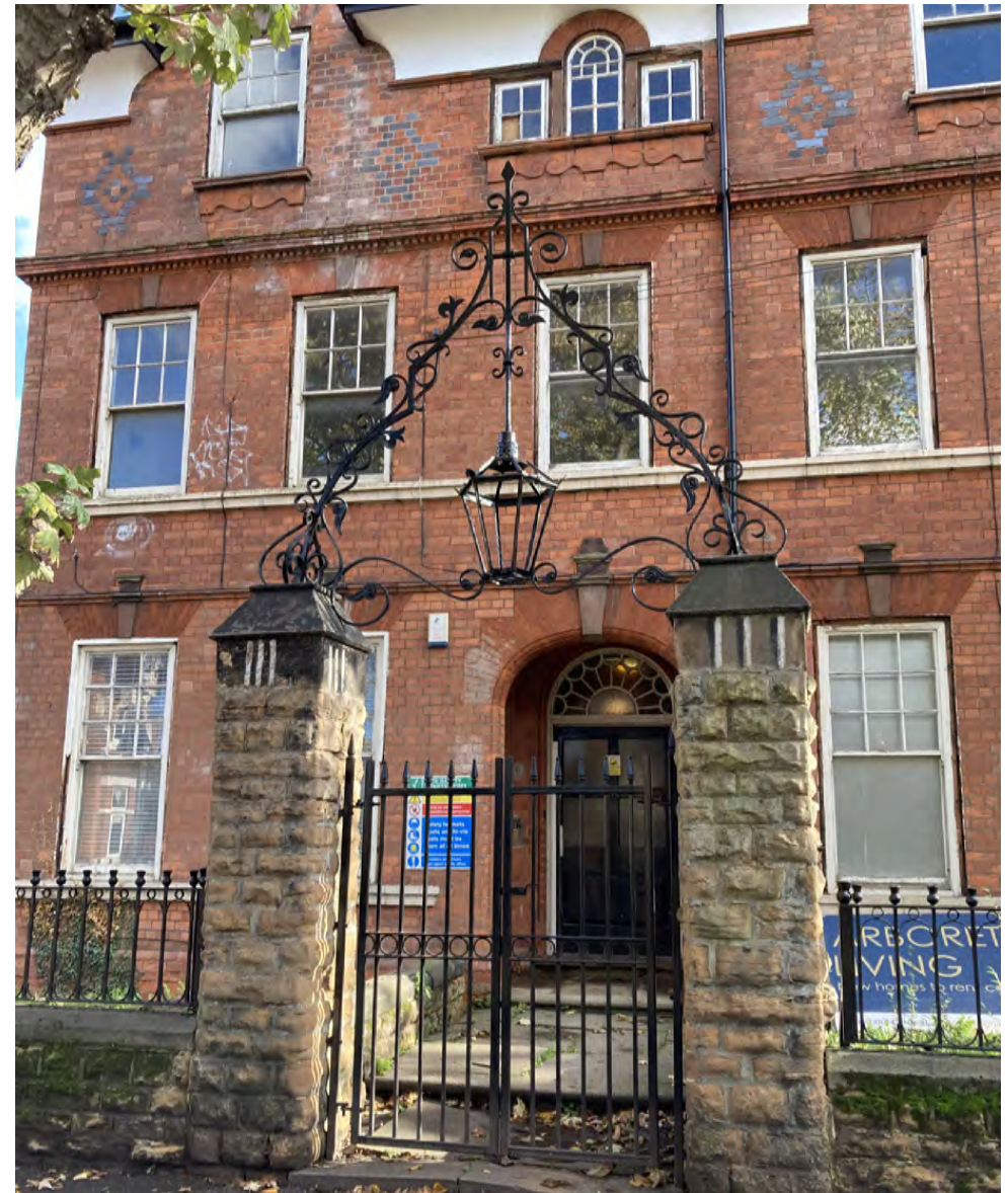
Photo right: No. 111 Forest Road - decorative ironwork arches
