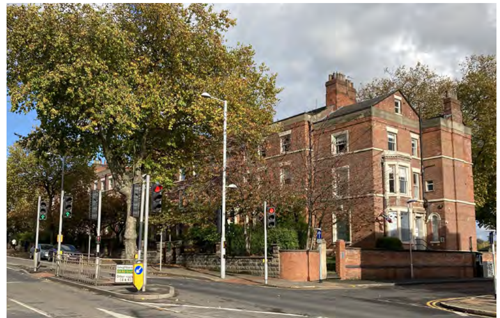
Photo below: Nos. 110 - 138 Mansfield Road
