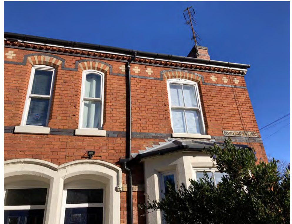
Photo below: Birkland Avenue - typical materials and detailing
