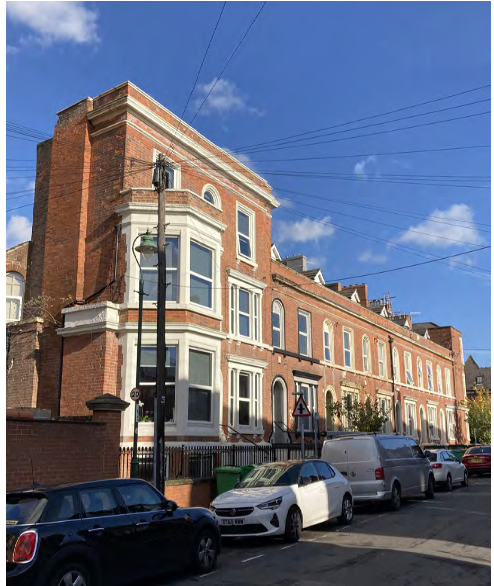
Photo right: Nos. 42-56 (Lang-Syne terrace) Burns Street
