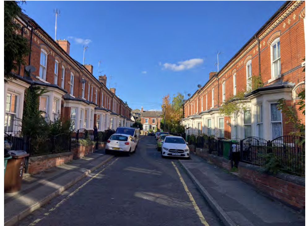
Photo below: Birkland Avenue
