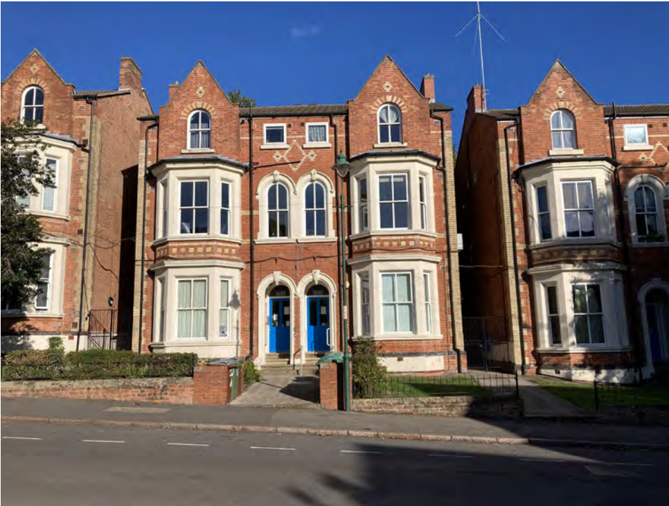
Photo below: Addison Street
