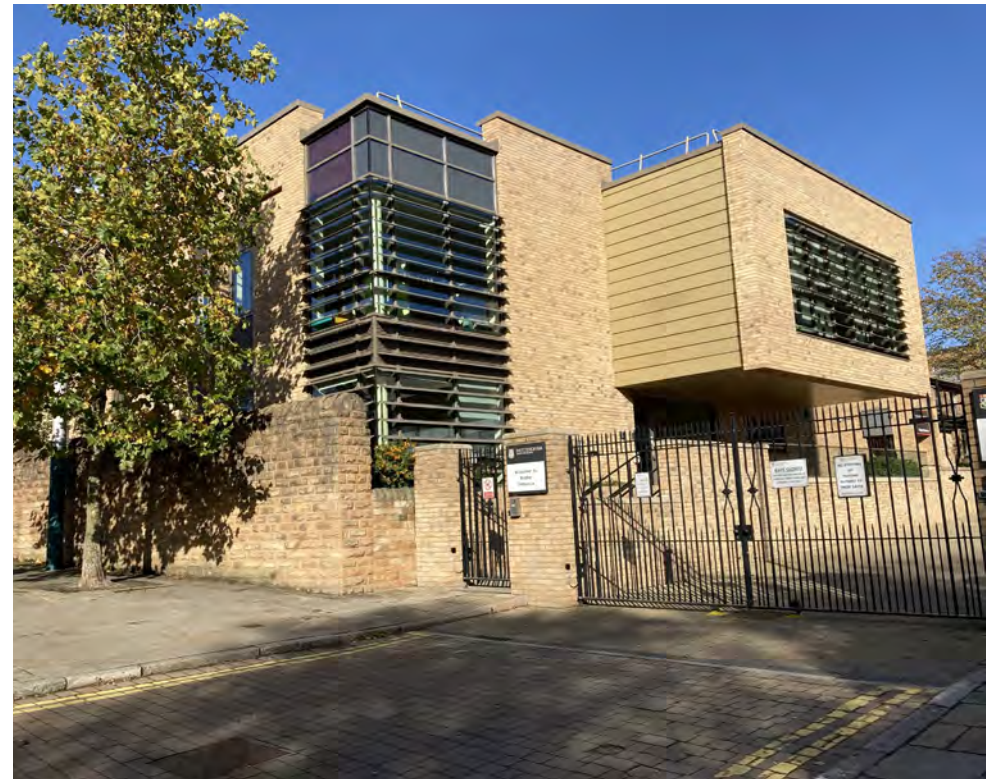
Photo right: Nottingham High School - Waverley Street
