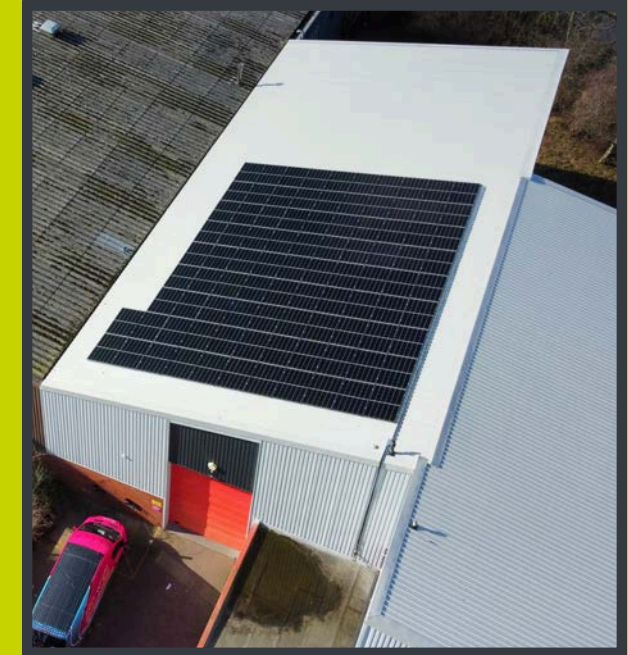
Solar panels at John E Wright
