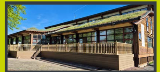
New decking at the St Ann's Advice Centre
