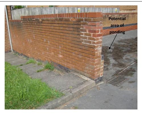
Figure 5: Brick wall potentially creating a barrier to flow at the north side of Daron Gardens. (N Facing)
