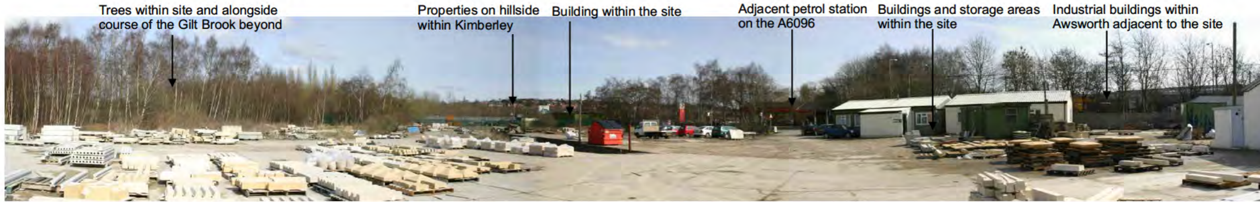
Photograph 2: view north east from within the site
