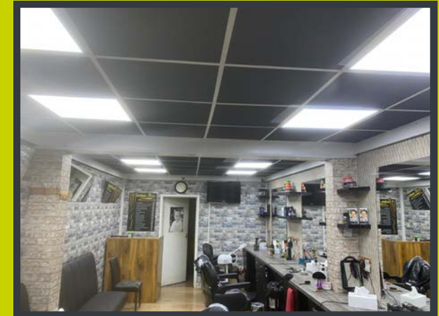
LED lighting and internal wall insulation at Blade Barbers
