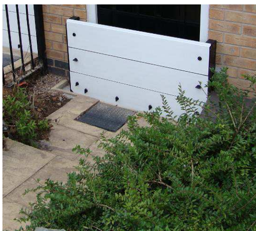
Figure 12: Flood boards installed following the storm in June 2010
