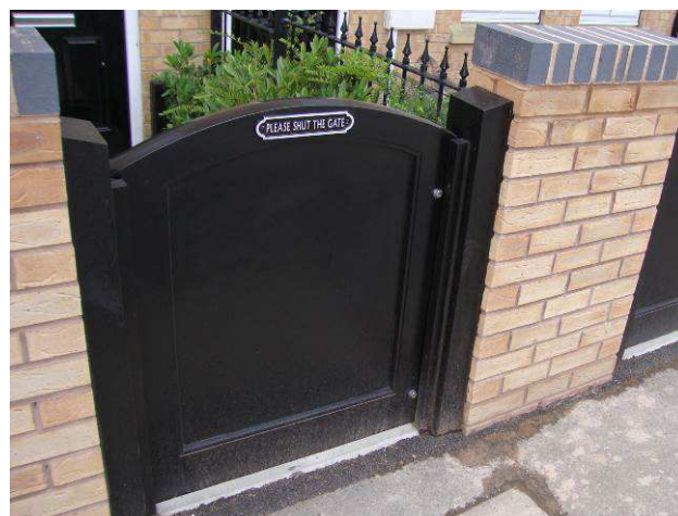
Figure 13: Flood wall and flood gates constructed in June 2011.
