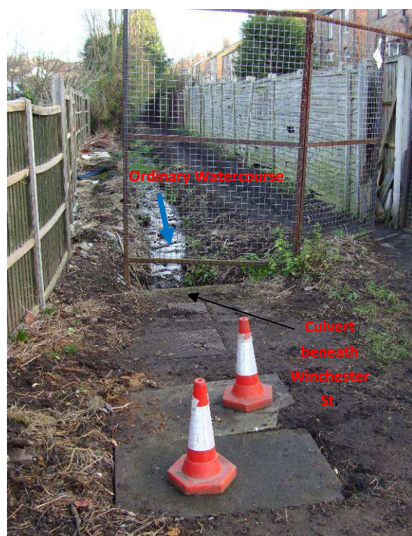
Figure 5: Ordinary watercourse that flows from Woodthorpe Grange Park behind Cavendish Vale and joins the public sewer network at Winchester Street. NE facing from Winchester Street.
