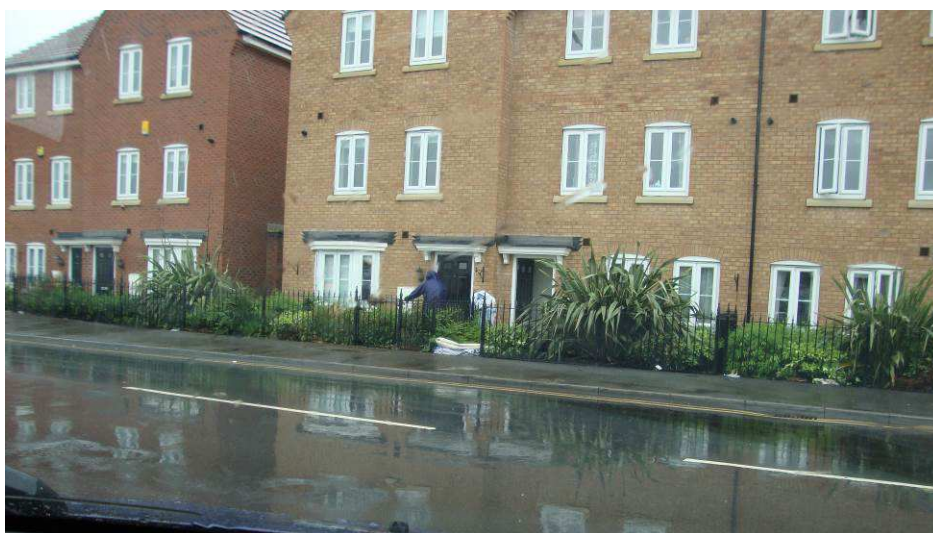
Figure 11: Haydn Road, west of Hucknall Road prior to the construction of flood walls.
