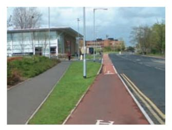
Figure 10.6 Cycle track transition to with-flow cycle lane (Patrick Lingwood)
