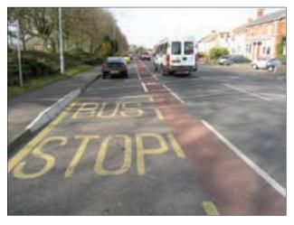
Figure 6.3 Cycle lane continued on the offside of bus stop and parking bays (Alex Sully
