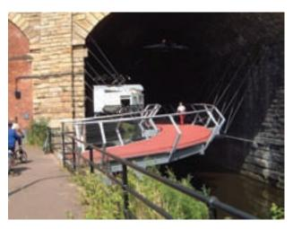
Figure 10.10 Cycle bridge suspended from a railway viaduct (Tim Pheby)
