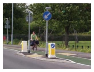
Figure 5.1 Cycle bypass ramped up to footway level (Patrick Lingwood)
