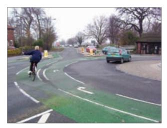
Figure 9.11 Roundabout with innovative cycle lane arrangement (Patrick Lingwood)
