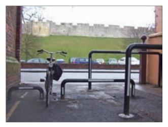
Figure 8.7 Barrier with wheelchair bypass (Tim Pheby)
