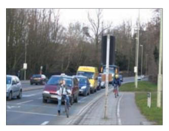
Figure 9.5 Cycle track bypass at a signalised T-junction (Patrick Lingwood)
