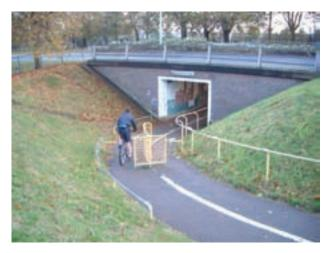
Figure 8.10 Barrier to reduce speed on approach to subway (CTC Benchmarking)
