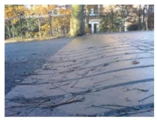
Figure 5.3 Flat-topped hump using pre-formed sinusoidal ramp face units (Tim Pheby)
