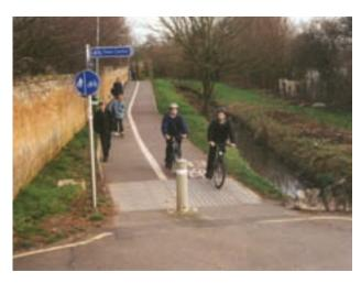
Figure 8.5 Bollard to prevent unauthorised car access (Alex Sully)
