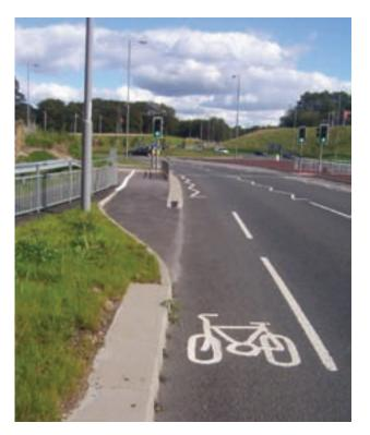
Figure 8.2 Smooth transition from carriageway to cycle track, Bingley. Note that the cycle symbol does not conform to diagram 1057 (see paragraph 3.3.2). (Tim Pheby)
