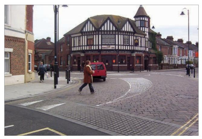
Figure 9.12 Mini-roundabout, raised junction and textured surfacing (Patrick Lingwood)
