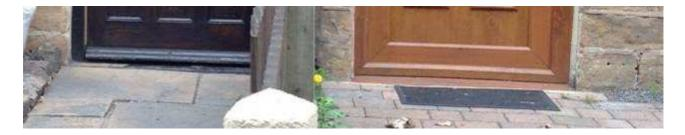
Figure 5: Low threshold of flooded properties on Bestwood Road allowing water to enter the properties.
