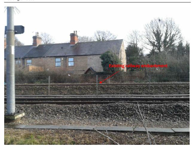
Figure 4: Existing railway embankment on the west side of Bestwood Road showing the height of the artificial barrier to surface water flow (Facing East)
