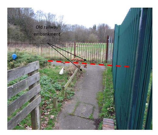
Figure 4: Old railway embankment (top of bank is marked by the red dashed line) forming artificial bund to the north of properties on Woolsington Close. Broxtowe Country Park is visible beyond the fence line.
